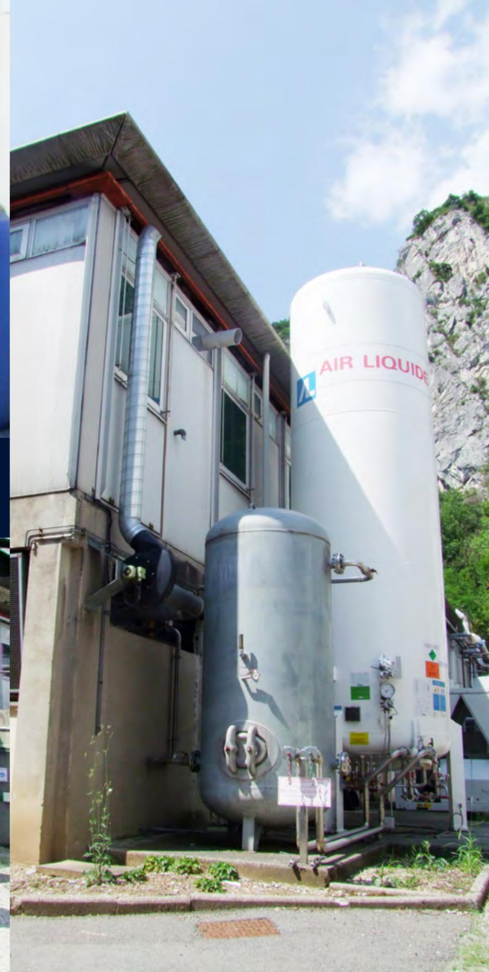
Tank air sec + azote liquide
